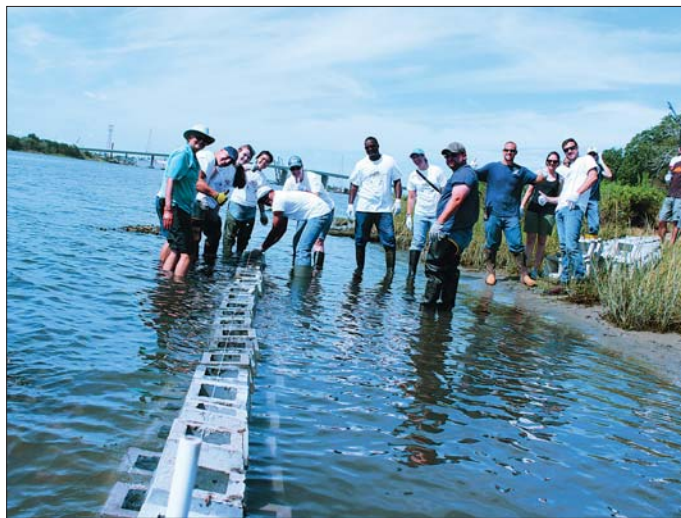
HRSD ORGANIZED VOLUNTEERS to install interlocking oyster blocks to augment a new oyster reef on the Eastern Branch. The wastewater authority constructed 118 "oyster bergs" using excess concrete.
